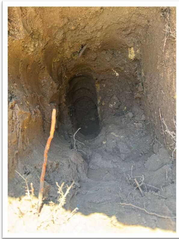
Photo 1: Trial pit showing foundation depth and sandy soil strata
